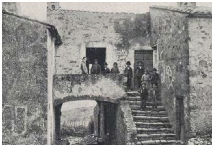
Figure 1. Exterior of the elementary school in Elmo Pianacce [from: Le Vie d'Italia XXXII, no. 10 (1926): 1093]
