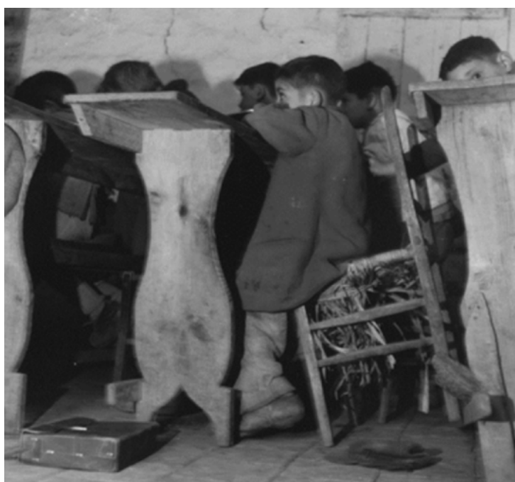
Figure 9. Interior of the elementary school in Jotta (1952)
