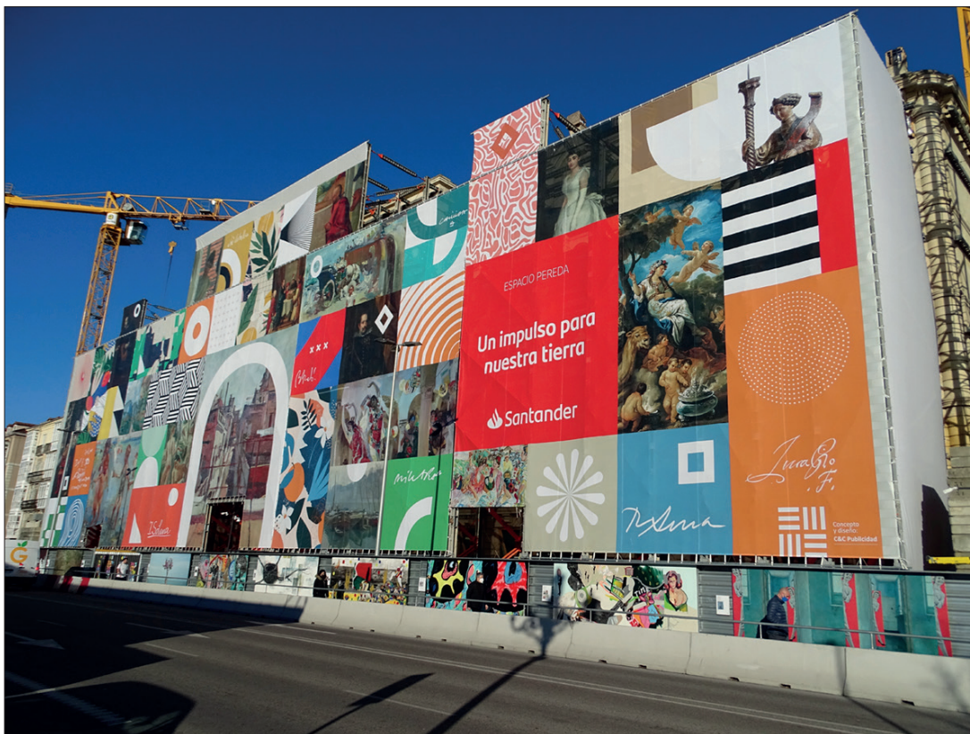
FIGURE 8. REHABILITATION OF THE MAIN HEADQUARTERS OF BANCO SANTANDER AS THE FUTURE ESPACIO PEREDA, SANTANDER. Source: Luis Walias Rivera
