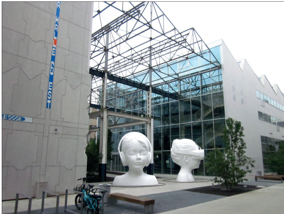
FIGURE 6. NANTES. INDUSTRIAL PREMISES HALLES ALSTOM IN HALLE 6 OUEST OF THE CREATIVE FACTORY WHERE THE ÉCOLE SUPÉRIEURE DE BEAUX ARTS DE NANTES-SAINT NAZAIRE IS LOCATED, AND ARTWORKS SET IN PUBLIC SPACE SUCH AS NATHALIE TALEC'S IN A SILENT WAY (2020). Source: Natalia Juan
