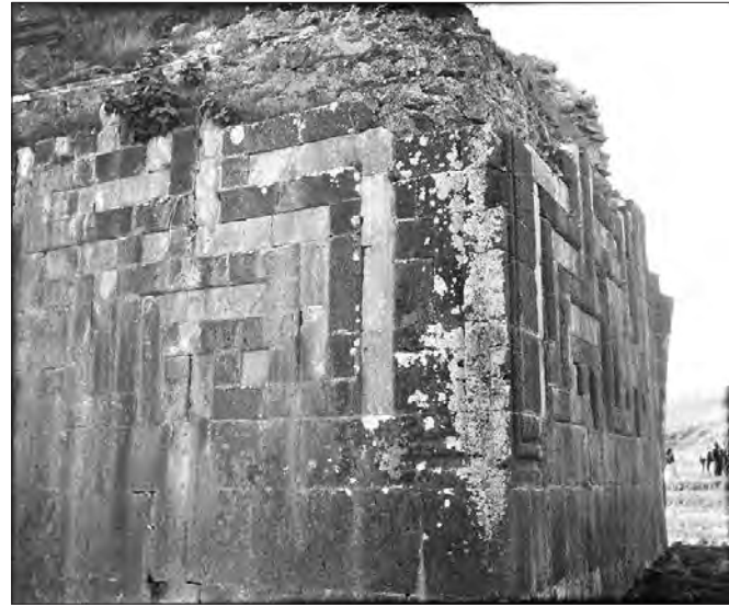
FIGURE 9. THE GEOMETRIC LIMESTONE AND BASALT FACING UP THE UPSTREAM SIDE OF THE SOUTHWESTERN PIER OF THE SURVIVING SPAN, AS PHOTOGRAPHED BY GERTRUDE BELL IN MAY 1909. The Gertrude Bell Archive, Newcastle University, M_090.
